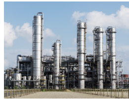
Oil and gas pipeline surveillance
